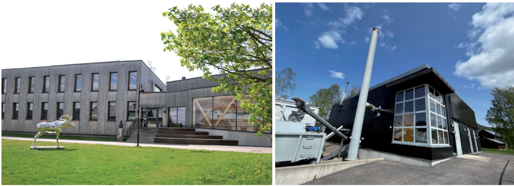
Figure 4. Left: Photo of the new administration and educational building at Evenstad. Right: The heating central at Evenstad (Photos: Anne-Lise Aakervik).
