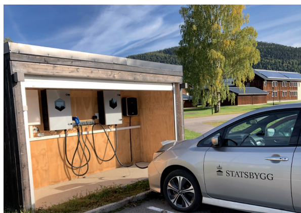
Figure 5. Left: Photo of the V2G equipment at Evenstad (photo: SINTEF). Right: Illustration of an example day with charging/discharging of two EVs, and its effect on the total power loads for Campus Evenstad.
