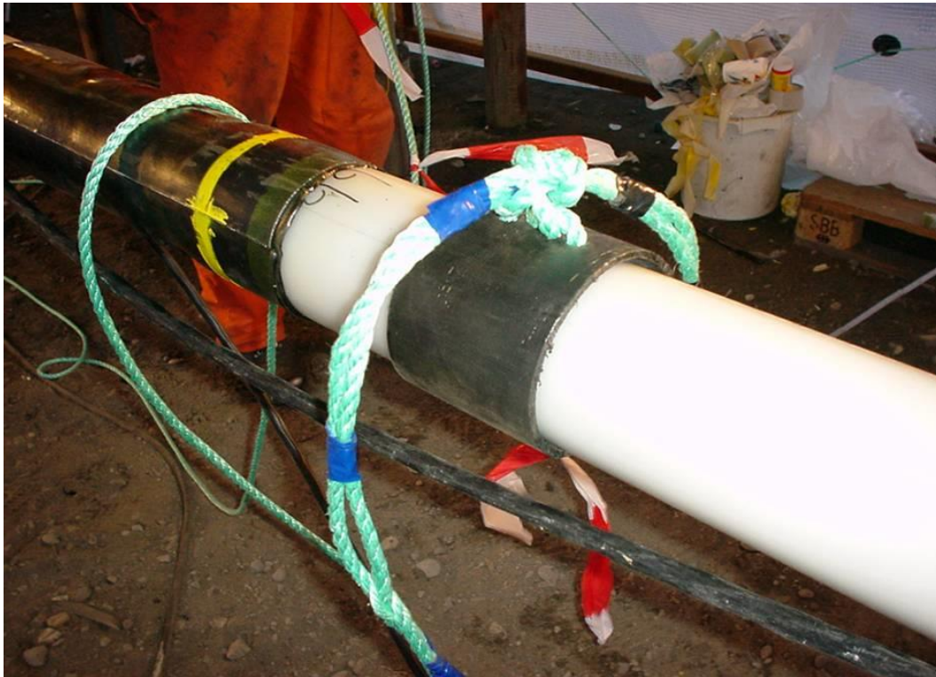
Figure A8: Electrically insulated pipe joint.
