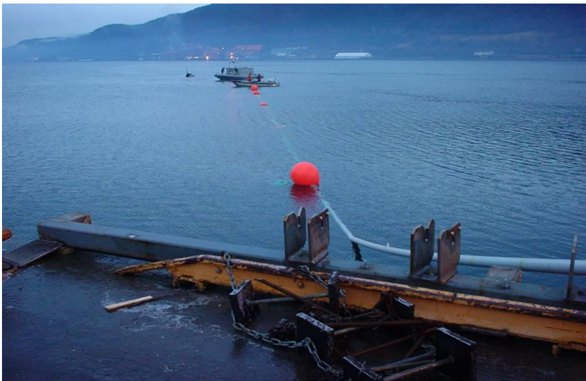
Figure A11: Floating the riser to position at the quay.
