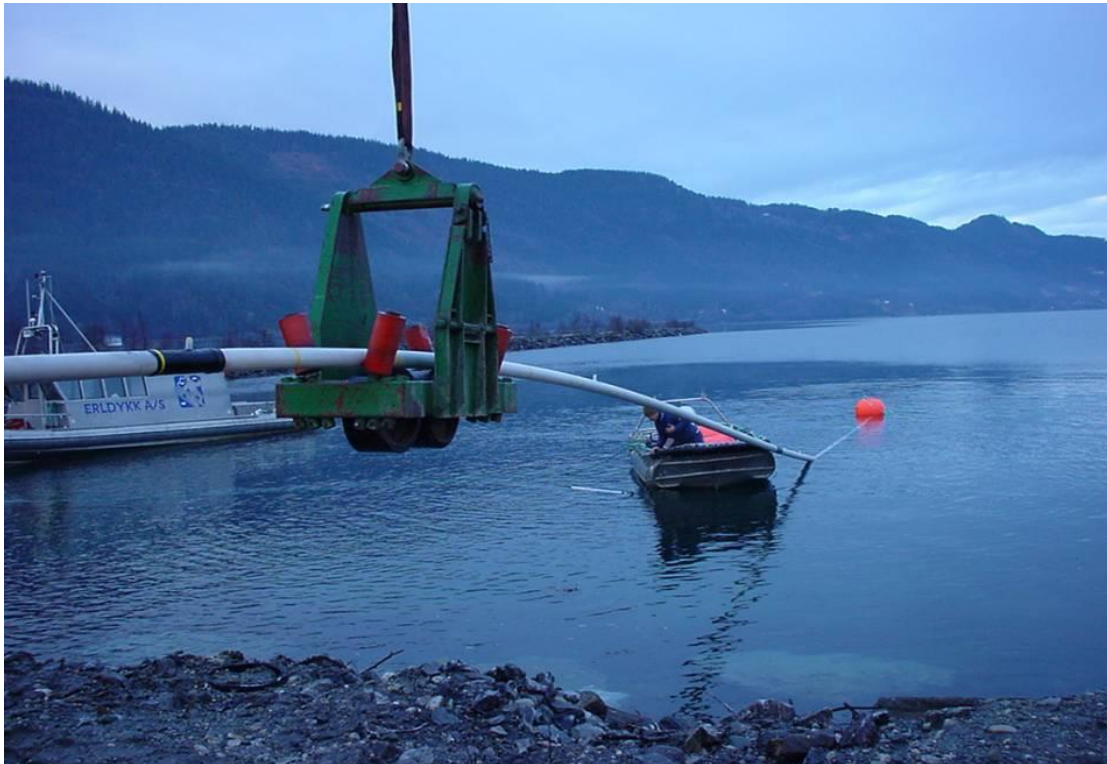
Figure A10: Raising the riser into seawater.
