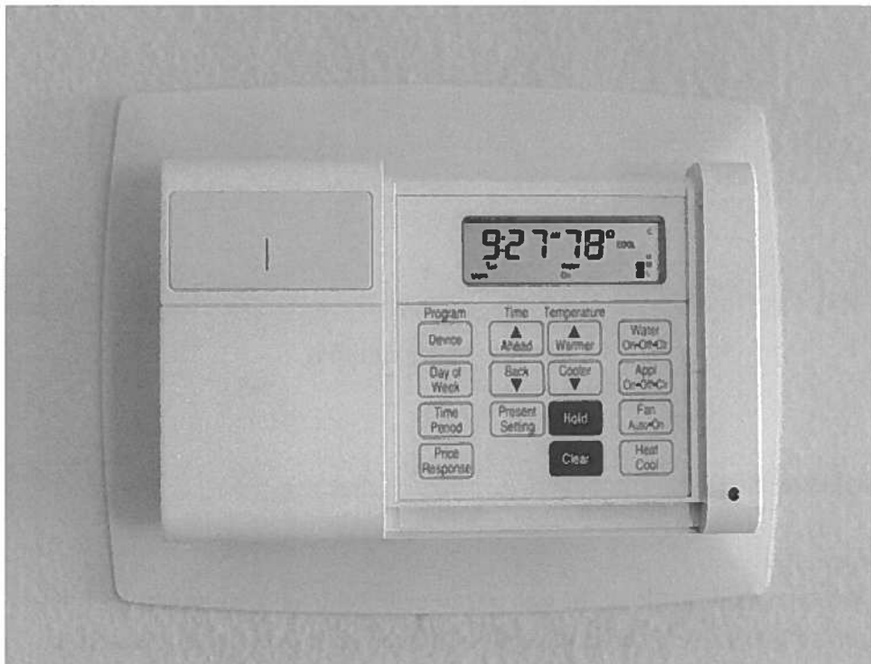
Figure A3: Smart Thermostat of Gulf Power.
