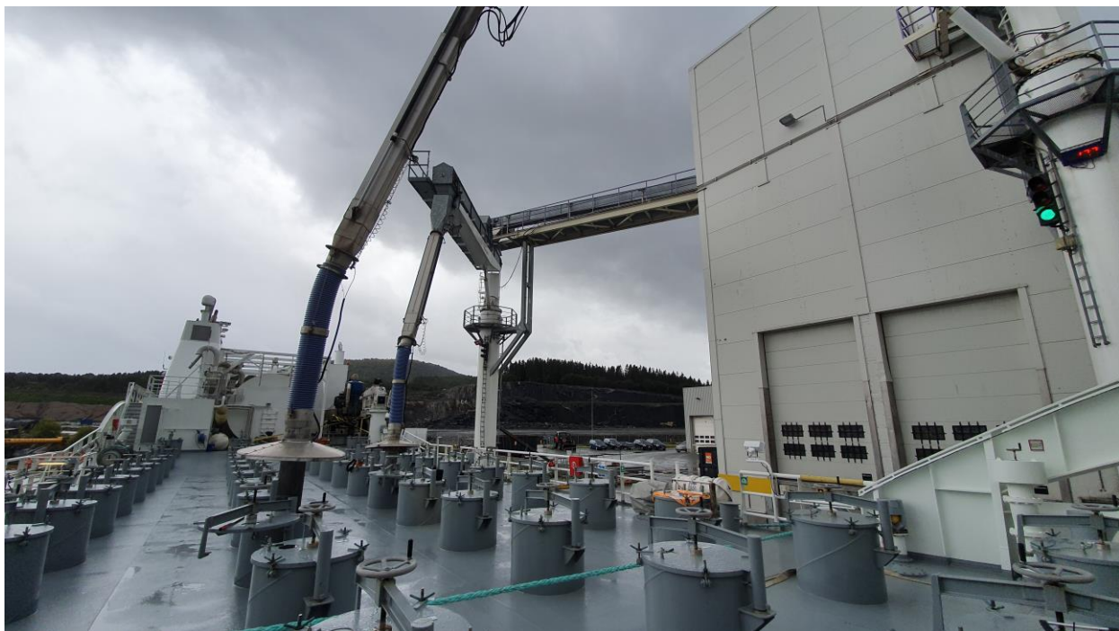
Figure 25: The two land cranes load feed into the ship silos at the factory quay.
