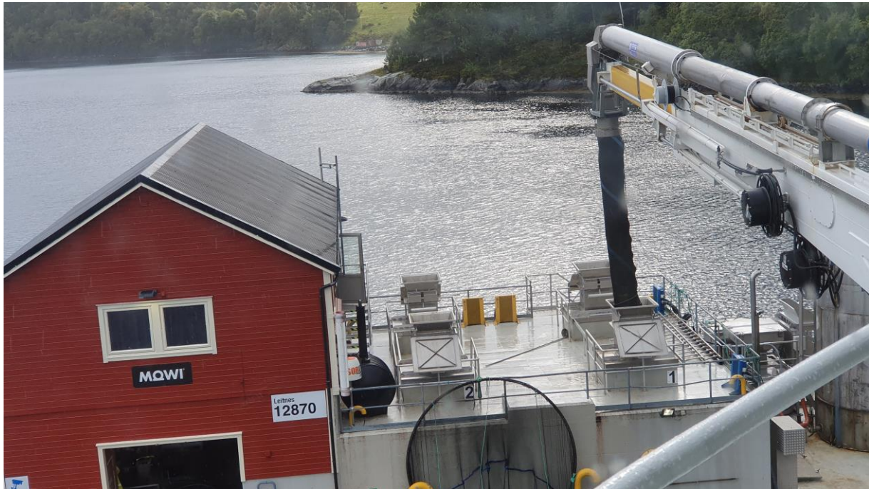
Figure 45: Offloading from ship to feed barge silo.
