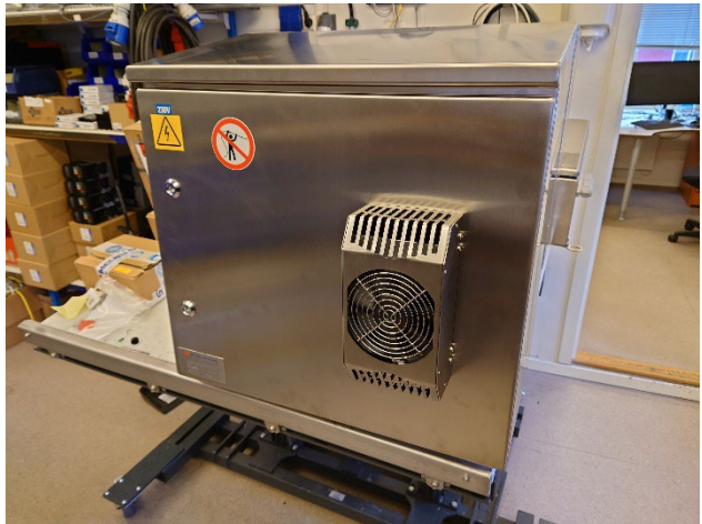
Figure 6: Thermoelectric cooler
