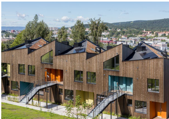
Ulsholtsveien. Source: Tove Lauluten/FutureBuilt
