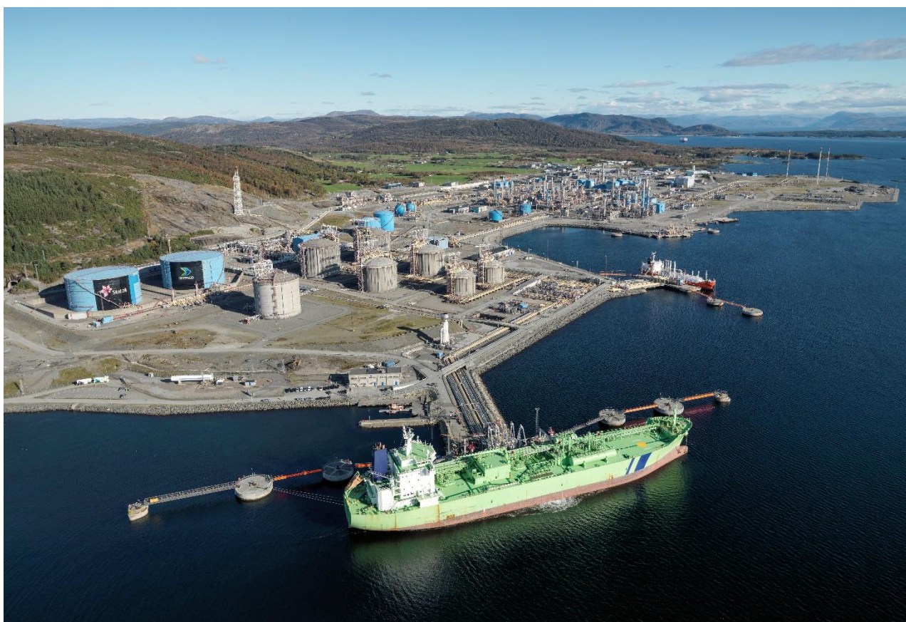
Figure 1-3: Overview of the Kårstø gas processing plant. Photo Markus Johansson /©Equinor.
