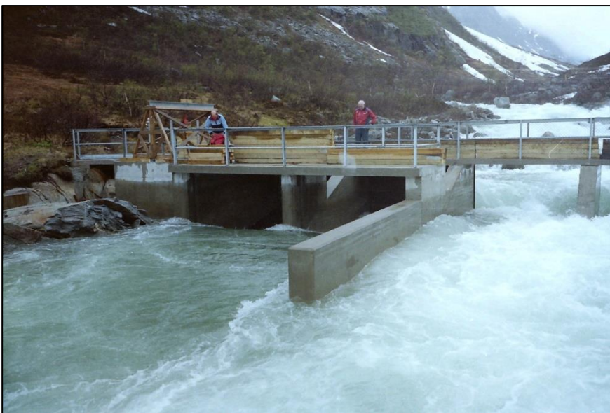
Figure 13: Intake at Otta secondary intake in Driva. modified Tyrol intake [28].
