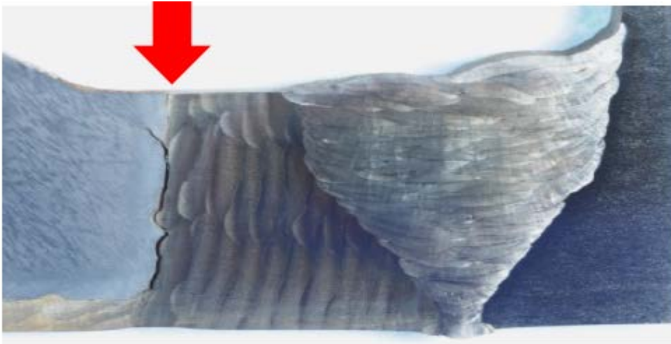
Figure 5 Picture of a hydrogen assisted failure of a HUB.
