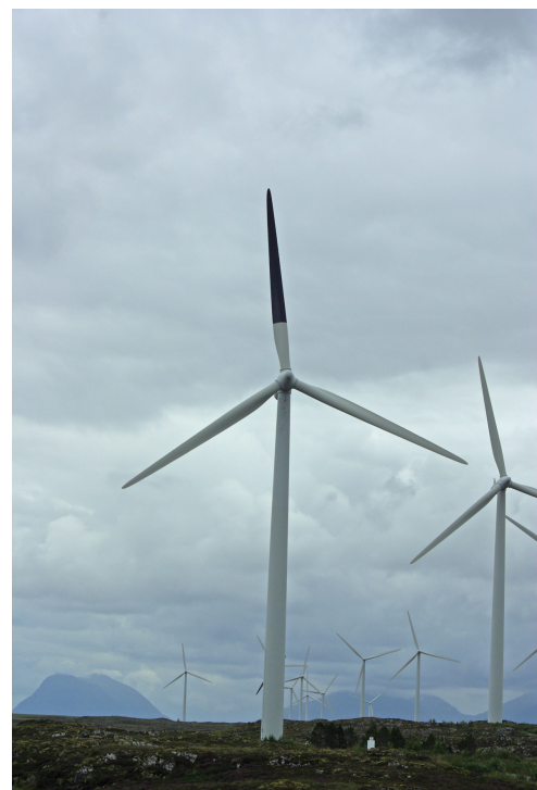
Figure 2. Wind turbine with rotor blade painted in black at the Smøla wind power plant, Norway. Image by May et al. 2020 [23] licensed under CC BY 4.0.
