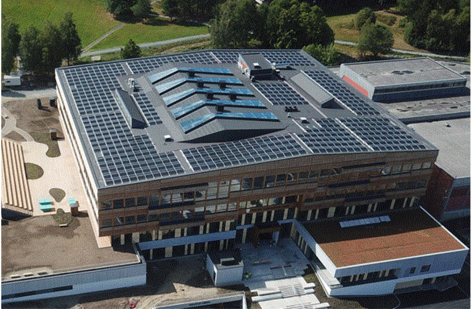
Figure 2. An overview of the PV installations located at Heimdal Upper Secondary School [Source: Trøndelag County Council].
