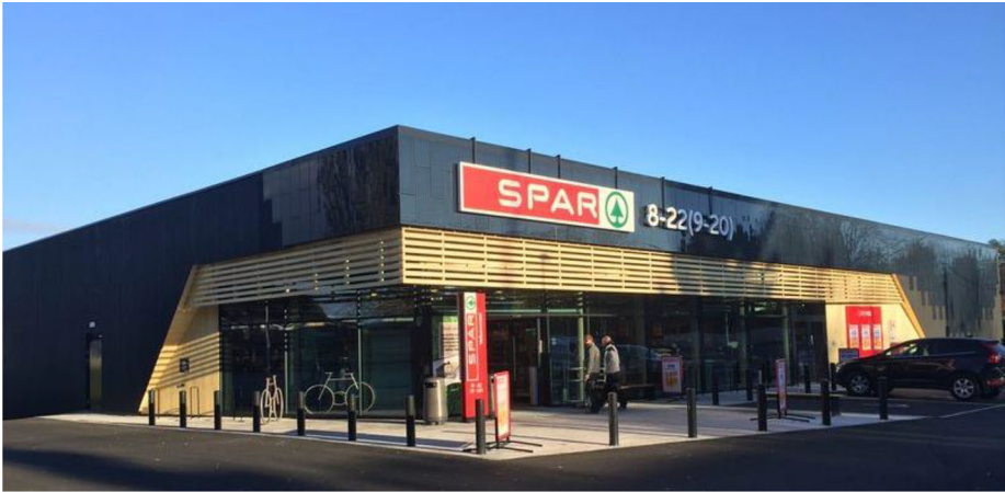
Figure 4. Spar Snarøya after completion, showing two of the facades with BIPV modules [Source: Norgesgruppen AS].
