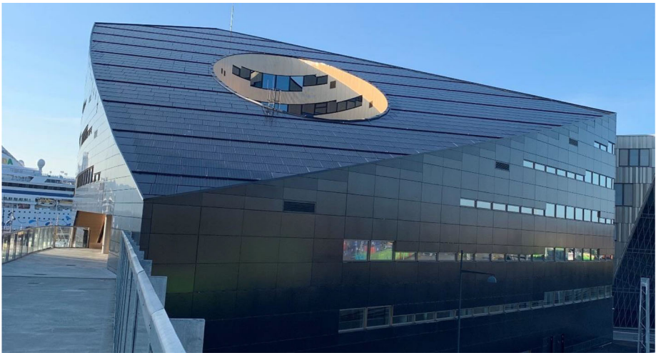
Figure 3. Powerhouse Brattøra after completion, showing parts of the south-facing façade in which parts of the façade is covered by BIPV modules and the roof with BAPV modules [Source: SINTEF].
