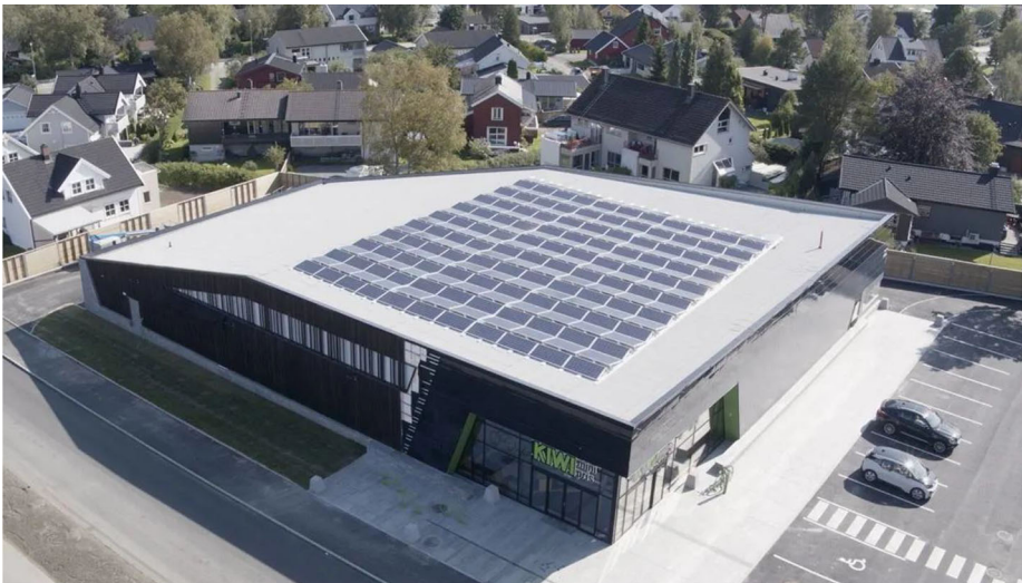
Figure 5. KIWI Dalgård after completion, showing two of the facades with BIPV modules and the roof with BAPV modules [Source: KIWI Norge AS].
