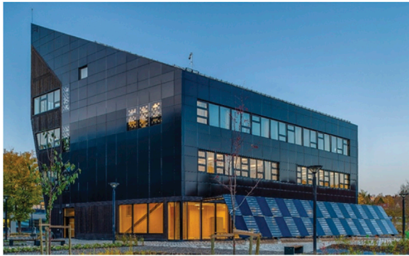
FIGURE 2 ZEB Laboratory: southern and western façade (© Photo: M. Herzog).
