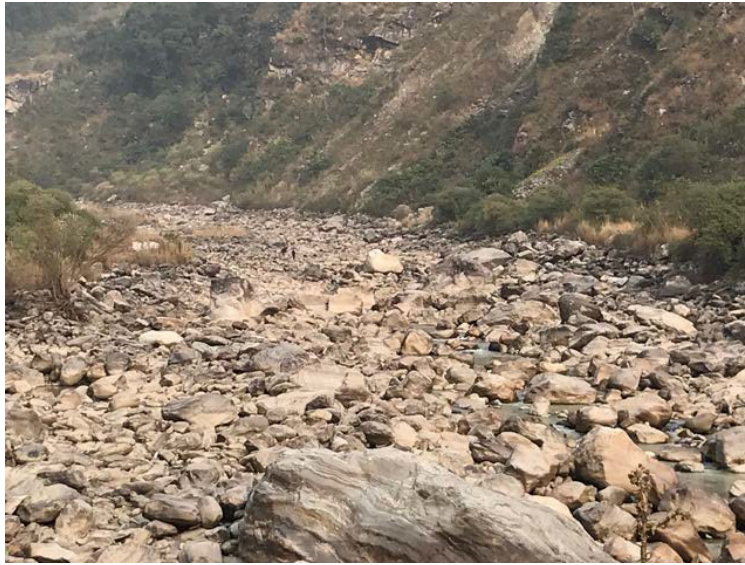
Figure 3. Diverted or bypassed reach downstream Upper Trishuli-3A HPP dam.
