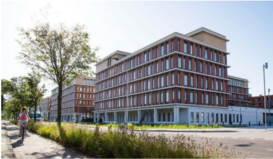
Figure 1. Exterior of the building
