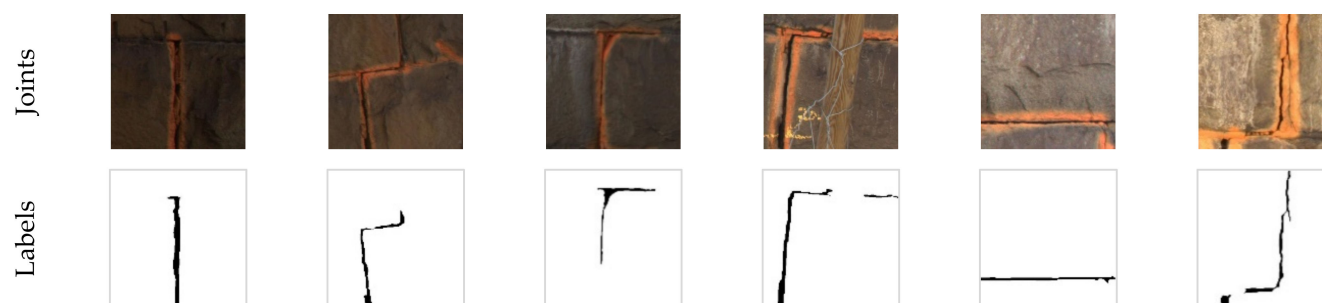
Figure 8. Examples of the prepared dataset used for pixel-wise damage segmentation.
