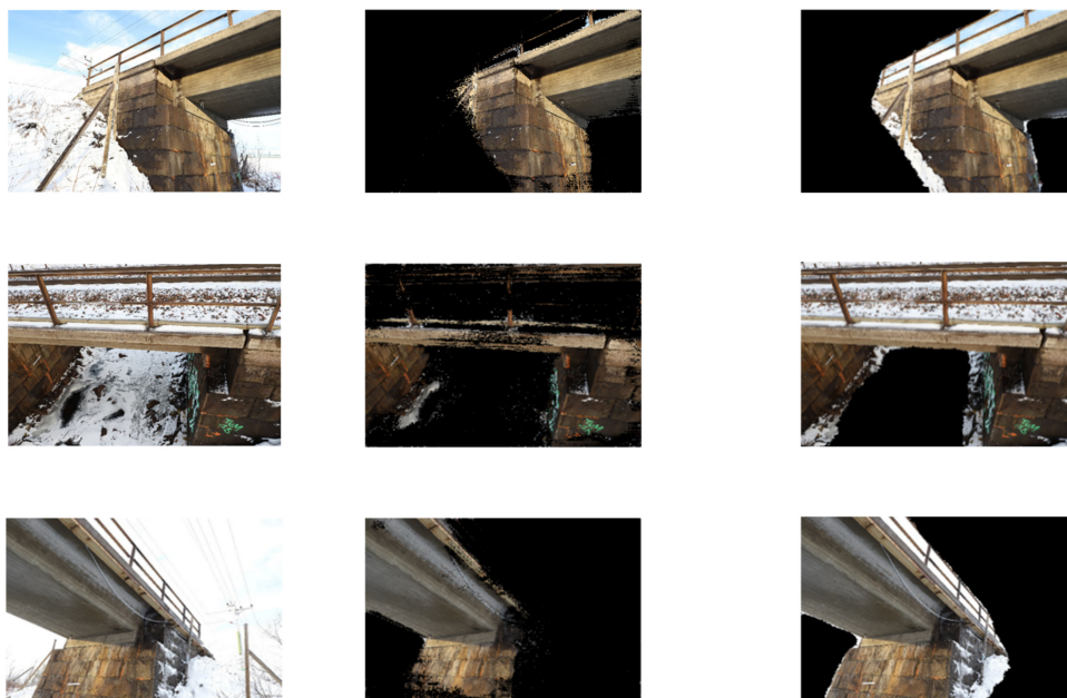
Figure 10. Detected bridge component by the studied CNNs.
