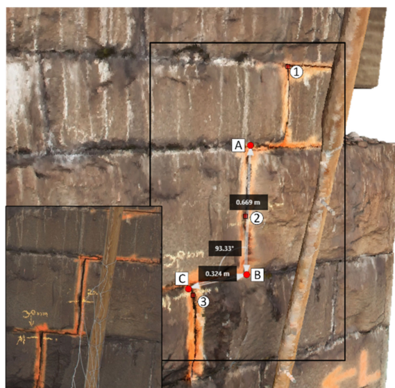
Figure 21. Damage measurement from TLS point cloud.
