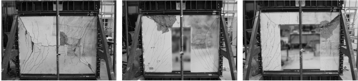
Figure 7: Crack pattern captured at failure of the unstrengthened specimens
