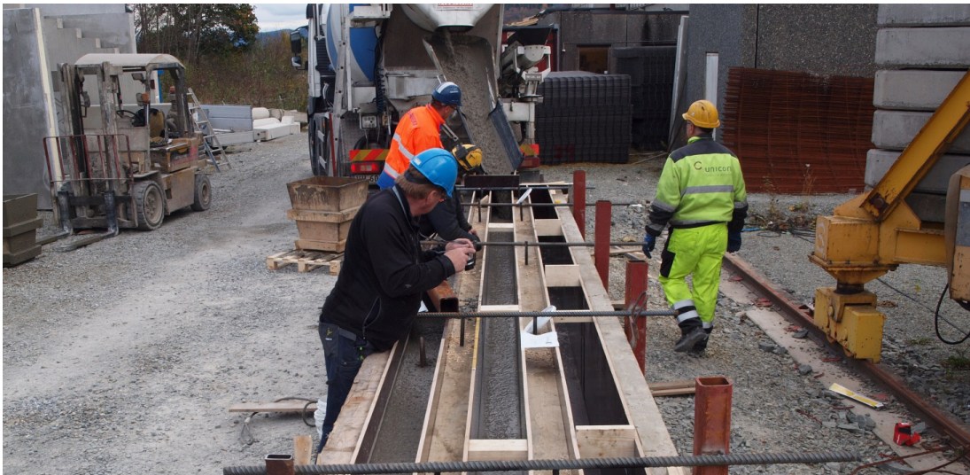
Figure 2 Casting of wall elements from truck gutter
