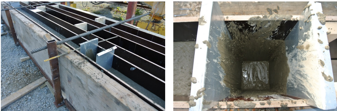
Figure 1 The wall elements with metal plates bounding the area for sampling.
