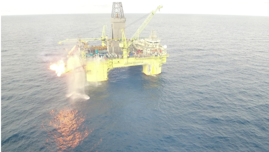
Figure 5.6 View from drone while it is near the center of the smoke plume during Flight 14. The curtain of water behind the flare is designed to protect the drill rig from the radiant heat emanating from the flare.
