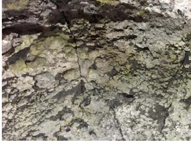
Figure 2.7. Pitting on the carbon cathode surface.
