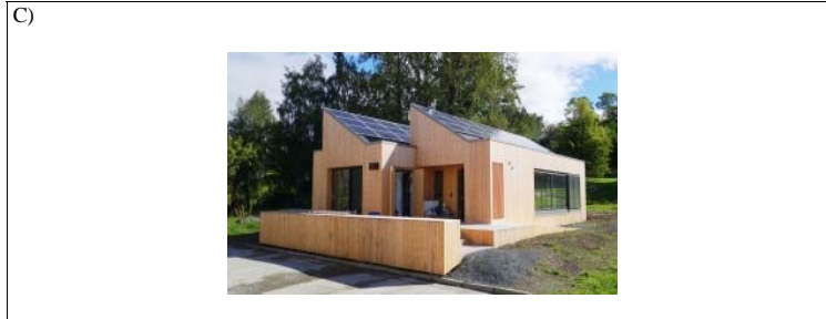
157 Figure 2 The roof mounted PV system design of the pilot buildings: A) Multikomfort (Kristian Edwards, Snøhetta) B) Skarpnes 158 (Skanska) C) Living Laboratory (Katrine Peck Size Lim)
