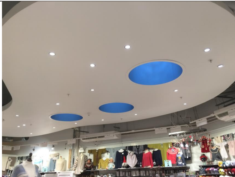
Figure 81. Picture of the ceiling with integrated spot lights and light tubes
