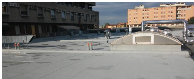
Figure 45. Roof painted using smart coatings.
