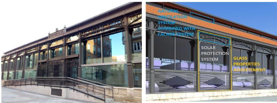
Figure 11. Multifunctional façade installed at the Mercado del Val
