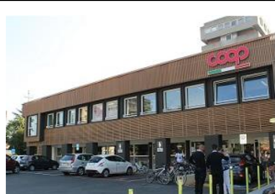
Figure 37. North-east facade after retrofit.
