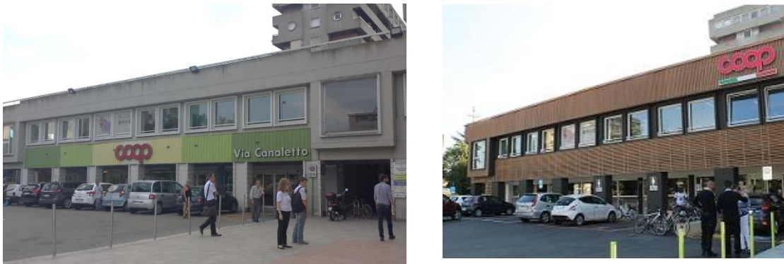
Figure 35. Coop Canaletto democase before (left) and after (right) the retrofit intervention.
