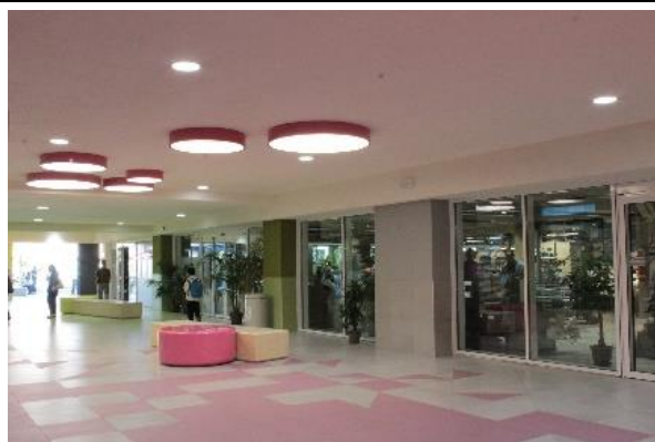
Figure 36. Glazed façade towards gallery after retrofit.
