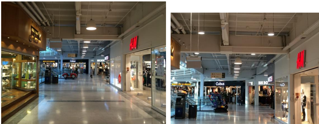
Figure 84. Initial situation and situation after retrofit (showing the GRL luminaire)
