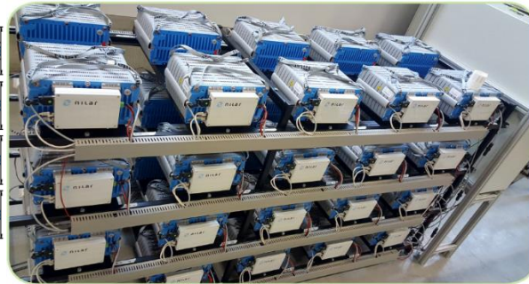
Figure 113. Battery energy storage system installed in the technical room in Marema' (Grosseto, Italy)
