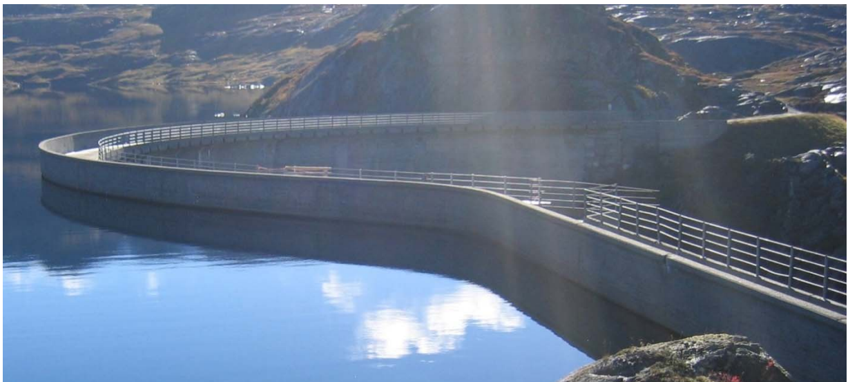
Figure 2. Photo of the Votna I dam (photo: J. Lindgård).
