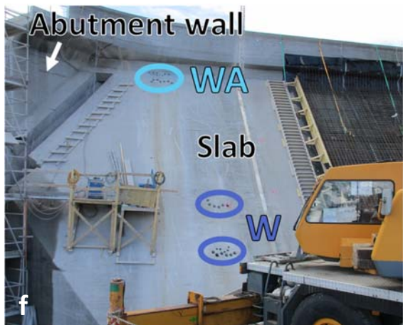
Figure 3. Photos of the Votna I dam at various locations: a) map cracking observed at the rail of the dam; b) map cracking observed inside the slab dam; c) presence of ASR gel in a bore hole in the dam; d) humidity inside the slab dam; e) aggregates visible on the surface of the concrete exposed to the reservoir (upstream face of the slab dam); f) upstream face after drilling of the cores and cutting of the blocks. May–June 2015 (photos a–e: G. Plusquellec; f: S.Å. Ekkje).
