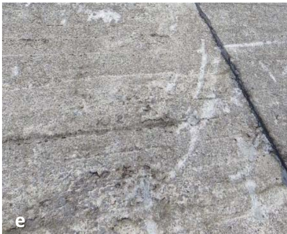
Figure 3. Photos of the Votna I dam at various locations: a) map cracking observed at the rail of the dam; b) map cracking observed inside the slab dam; c) presence of ASR gel in a bore hole in the dam; d) humidity inside the slab dam; e) aggregates visible on the surface of the concrete exposed to the reservoir (upstream face of the slab dam); f) upstream face after drilling of the cores and cutting of the blocks. May–June 2015 (photos a–e: G. Plusquellec; f: S.Å. Ekkje).
