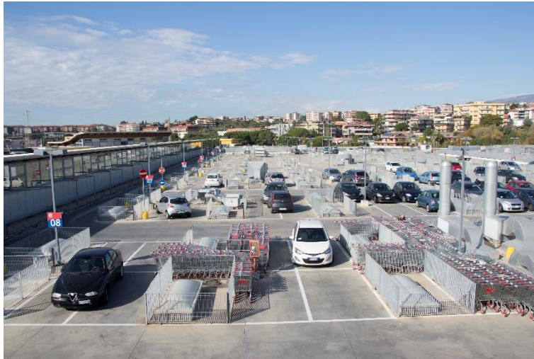
Figure 171. View of the parking on the roof.
