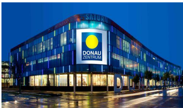
Figure 8-2. North-West view of BT7
