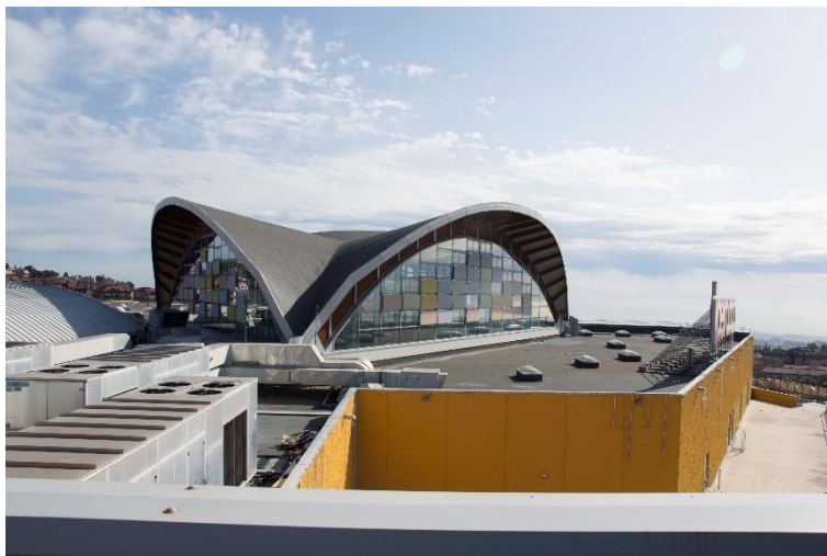
Figure 173. Skylight over the southern stairwell shaft.
