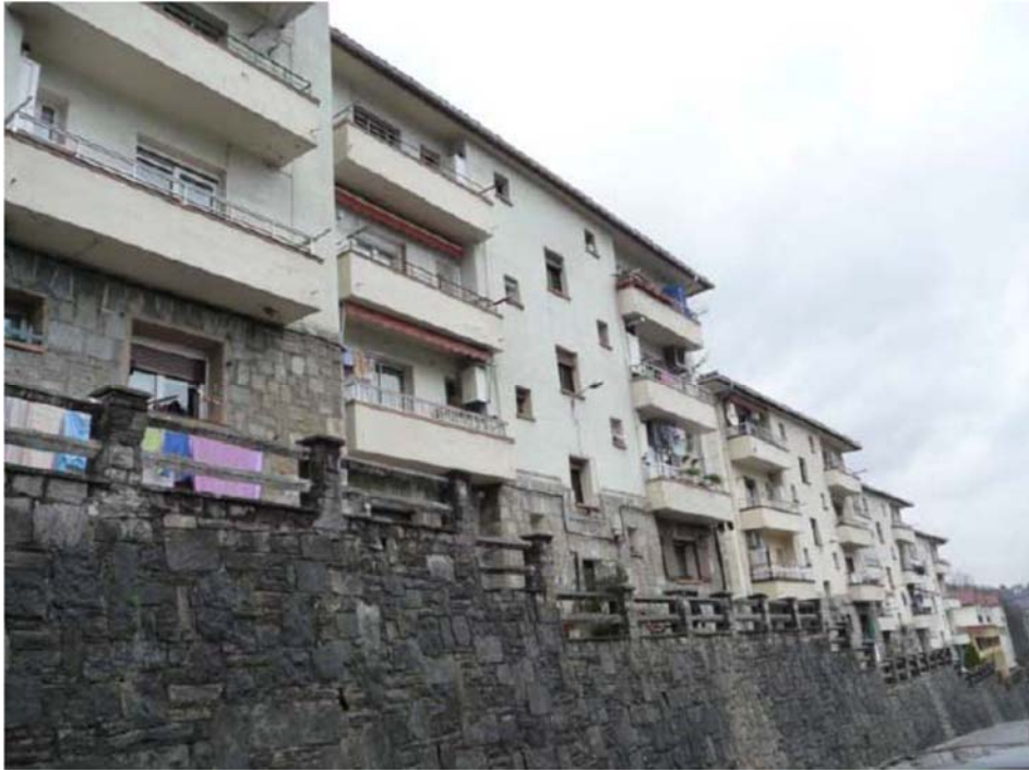
Figure 3.2 District Of Zerukoia (Ermua): 250 dwellings in fifteen blocs of flats (Ground floor + 5, 6 or 10 storeys)
