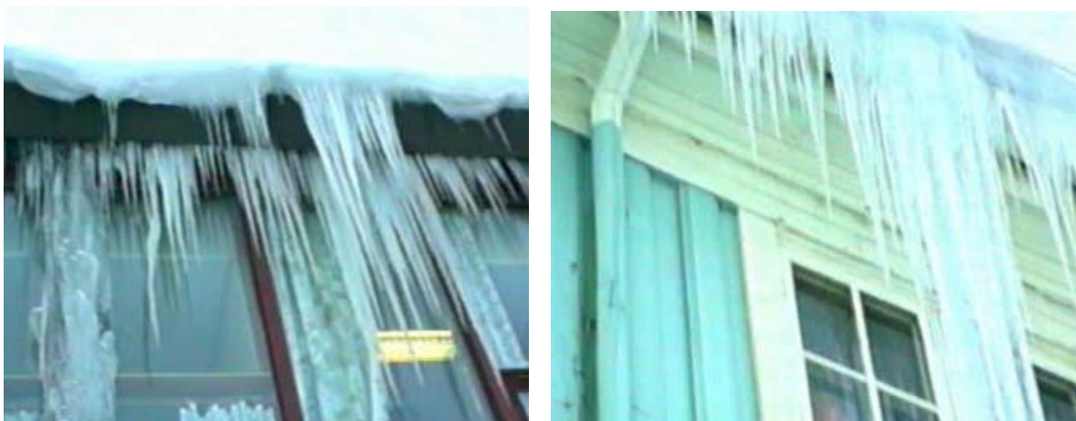
Figure 4. Large icicles in front of the glass facade of a school building, covering the windows and representing a hazard to the children (left) and large icicles blocking the window and representing a hazard to the people below (right). (Photo: SINTEF Building and Infrastructure).
