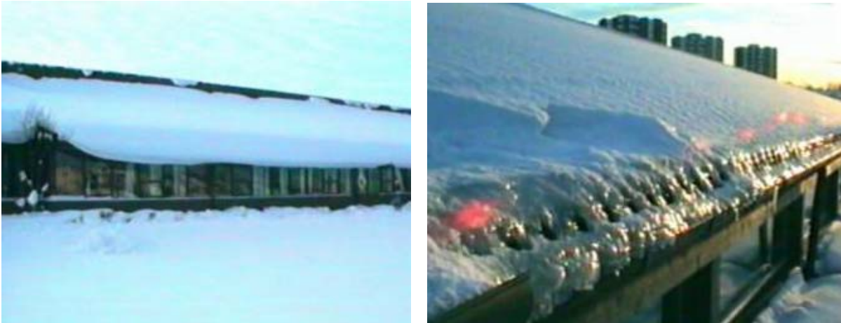
Figure 2. Snow hanging from roof and covering the glass facade of a school building (left) and rain gutter at the eaves completely full of ice (right). (Photo: SINTEF Building and Infrastructure).
