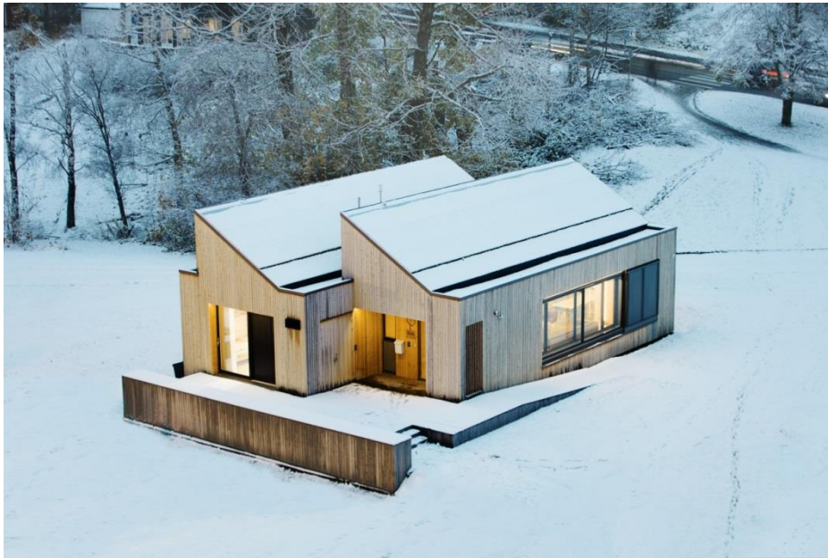
Figure 1.2 Picture of the ZEB Living Lab on the Gløshaugen campus, NTNU (image by ZEB).
