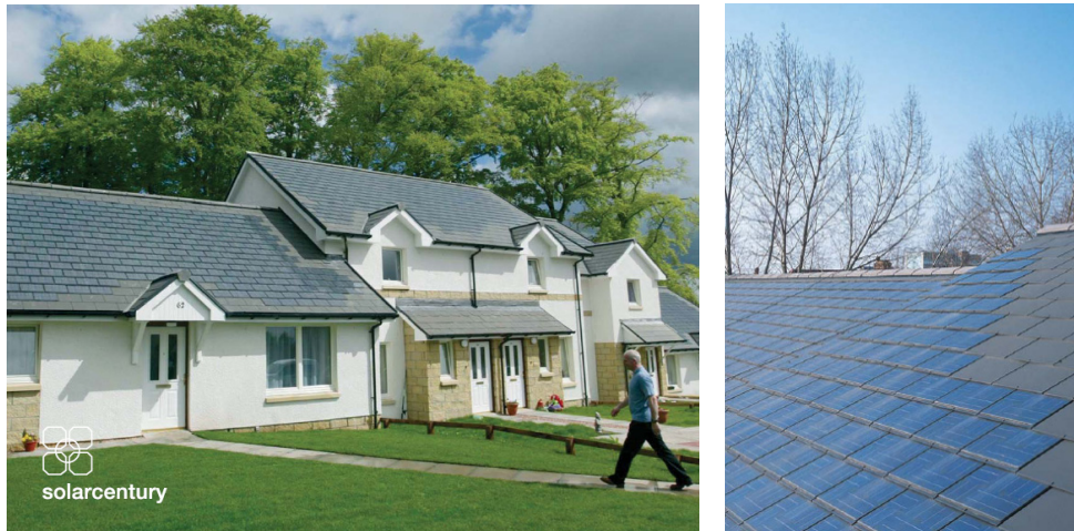
Figure 26. Example of building integrated photovoltaics (BIPV) (Solarcentury 2008).
