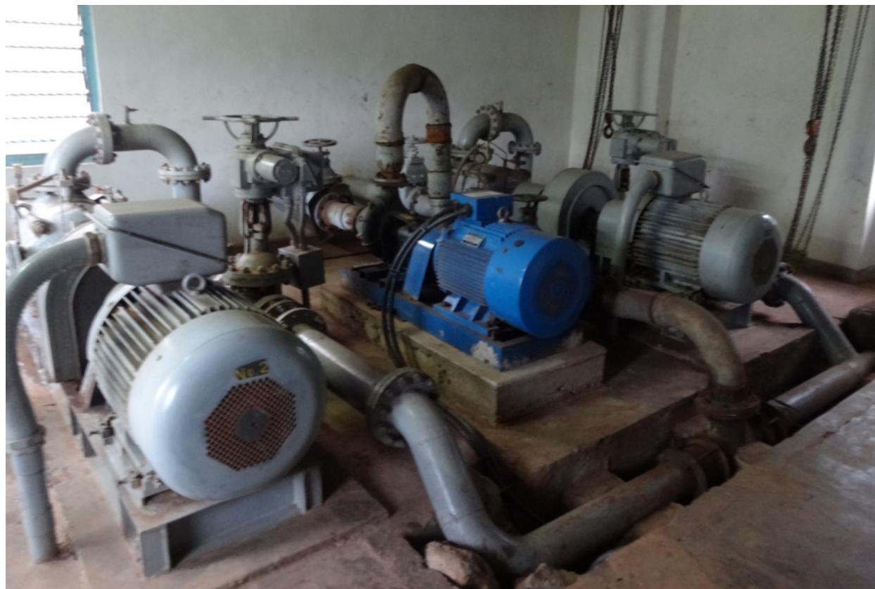
Figure 2: Pumps in the pump house for the water supply system in Taveta city
