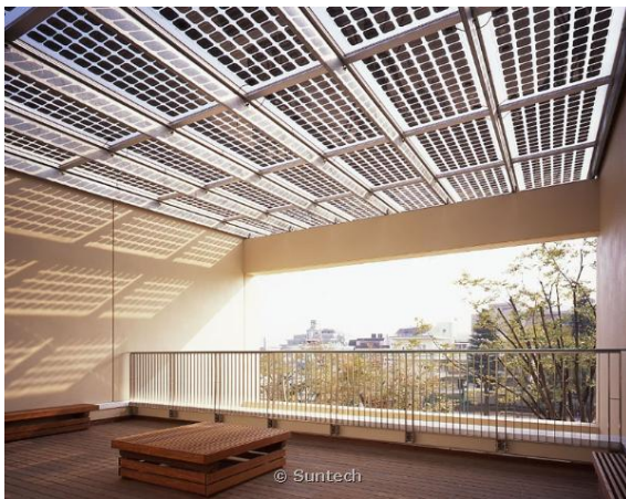
Figure 4: Glass ceiling with transparent BIPV modules (Global Energy Network Institute 2009).
