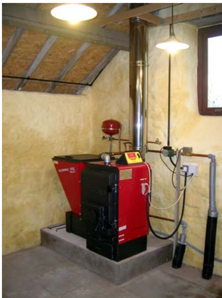
Fig 5.7 Pelletskjel m/ lager. Kilde: The Harman Accentra Pellet Stove http://pelheatblog.com/2008/11
