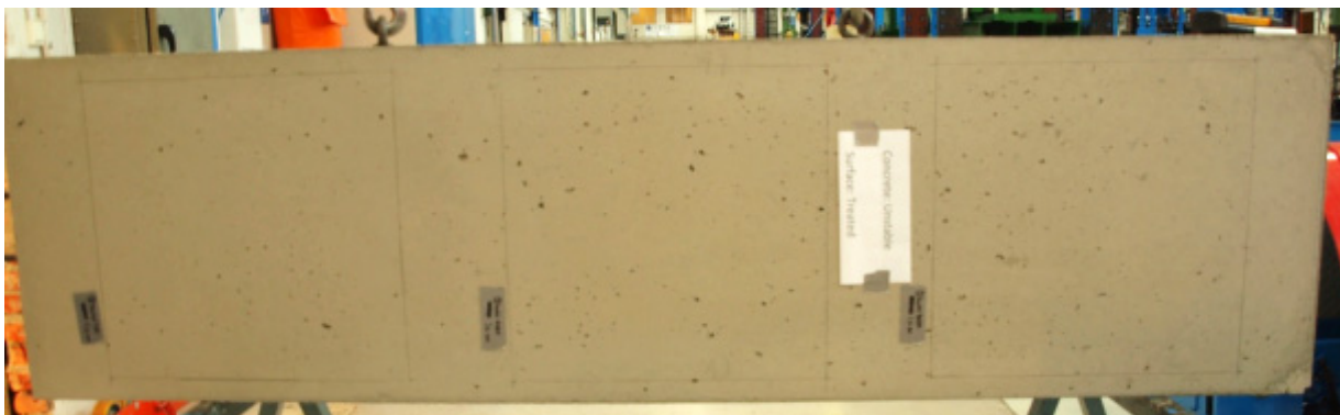
Figure 9: Positioning of the bottom, middle and top zone of the surface of a wall element. (left to right)
