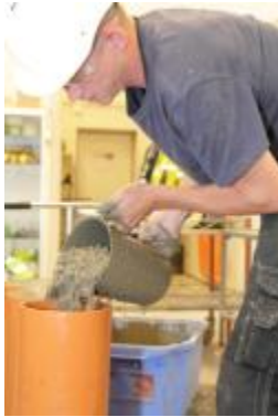
Figure 8: Filling of the PVC columns with fresh concrete
