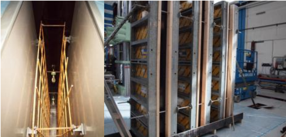
Figure 1: The reinforcement and formwork for the three wall elements.
