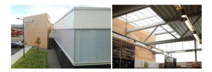
Fig. 5. The Rama 1000 supermarket at Kroppanmarka with 220 m<sup>2</sup> aerogel glazing panels [19, 21].
