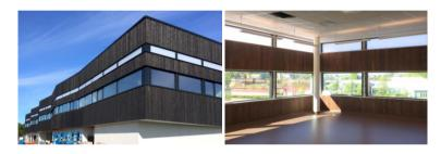
Fig. 6. Levanger primary school, Norway. The entire second floor has built with two glazing systems: aerogel glazings for upper windows and normal clear glass glazings for low windows [21].
