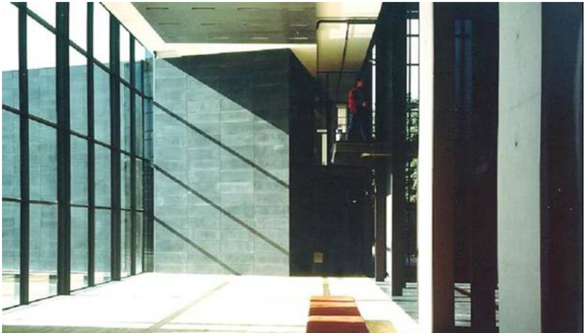
Figure 6.12: Heavy materials, concrete and stone, give thermal mass which even out temperature swings. Picture from the headquarter for E. Pihl & Søn in Lyngby, Denmark. Office building from 1994. KHR AS Architects. ( http://www.khras.dk/Projekter/Kronologisk?g=60 )
