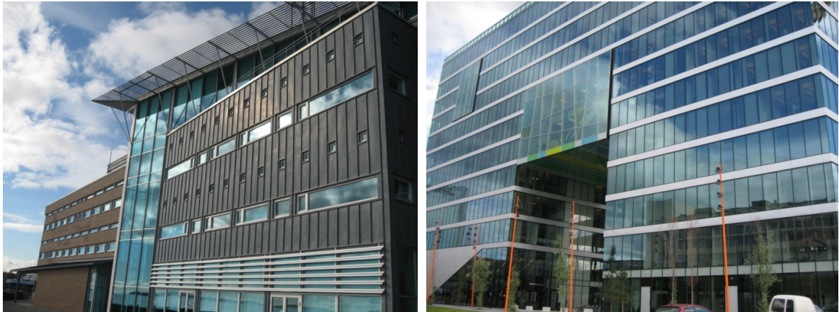
Figure 6.2: Examples for the use of glass in the facade (left: example of less use of glass; Senter for Marint Miljø og Sikkerhet in Horten, right: example of more use of glass; PriceWaterhouseCooper i Oslo, Photos: Sintef Byggforsk)
