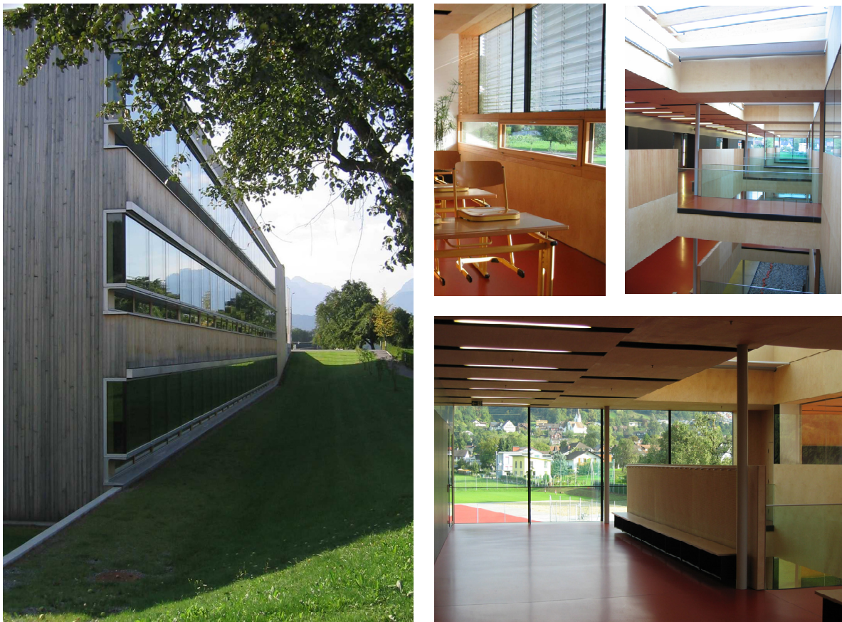
Figure 6.10: Schule Weiler i Vorarlberg, Østerrike. University with passive house standard. Windows on east and west orientated facades are divided into two parts. The lower part allows direct view to the outside if the shading system is down. The picture on the upper right shows the bridges to the classrooms. The inner part of the building is daylighted from skylights. The open areas connect the ground floor with the skylights. The lower right picture shows the entrance area with wardrobe. Window areas are oriented towards north and do not need solar shading. Architect Dietrich Untertrivaller. Photos: SINTEF Byggforsk.
