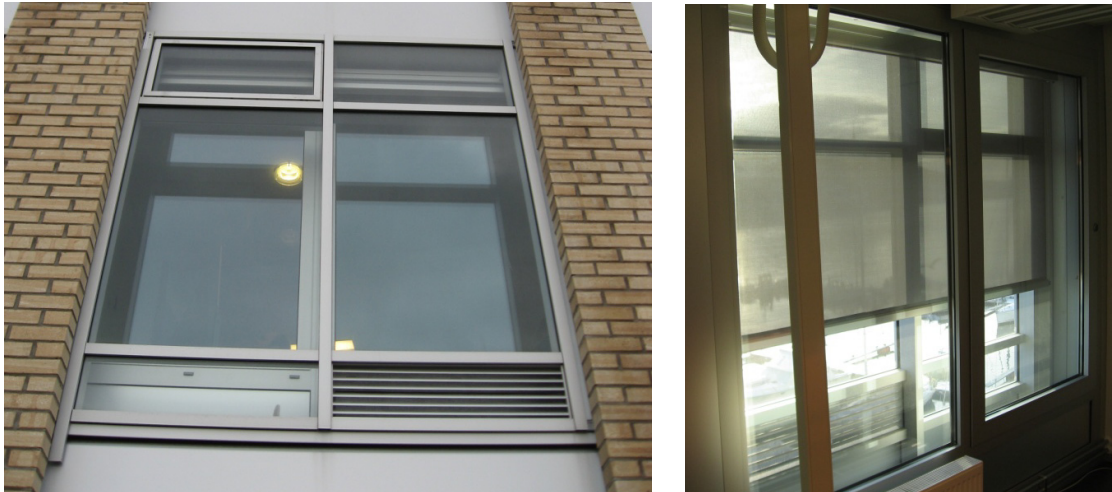
Figure A.4: Double facade with fixed opening below and controlled opening at the top (left) and solar shading in the cavity (UN-grid building in Arendal, Photos: SINTEF Byggforsk)
