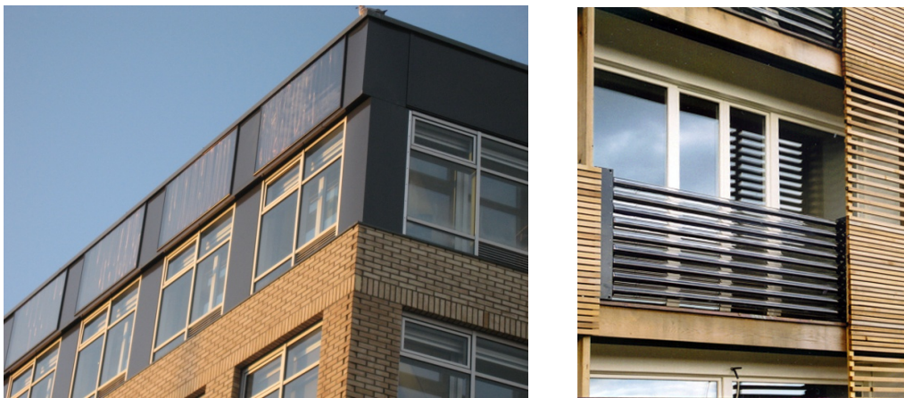
Figure A.11: FPC integrated into the facade (FN Bygg, Photos: SINTEF Byggforsk), ETC can also be used as facade elements, f.e. as railings in balconies.
