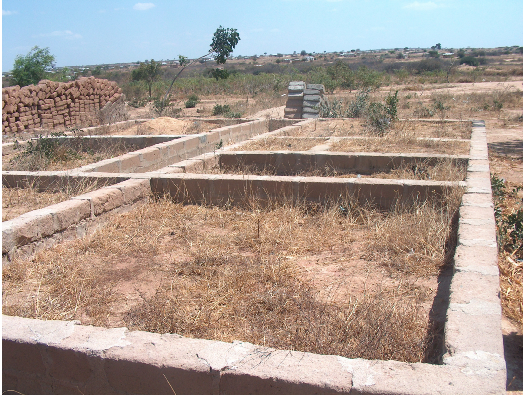
Fig. 2.3 Construction at foundation level
