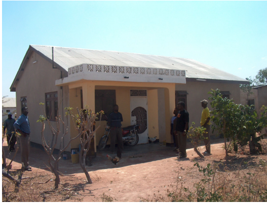
Fig. 2.6 A completely built 75m 2 House
