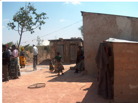
Fig. 2.5 External shower and pit latrine.
