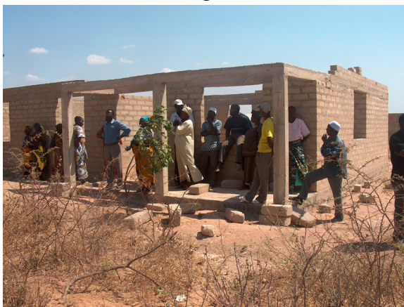
Fig. 2.4 Construction using stabilised soil blocks
