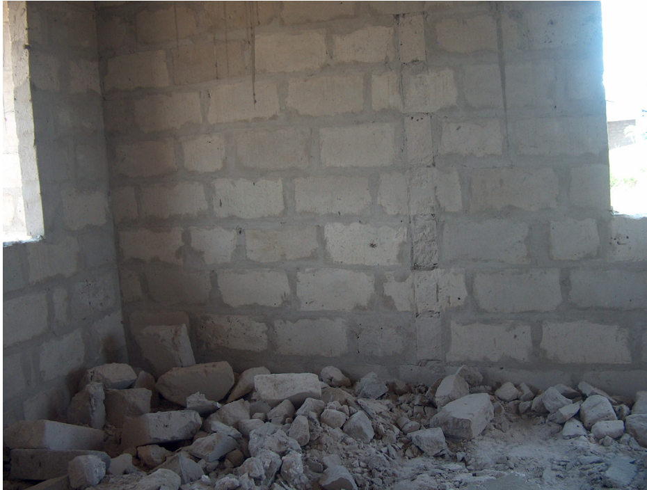
Fig. 2.12 Demolished Wall Living Room/Kitchen
