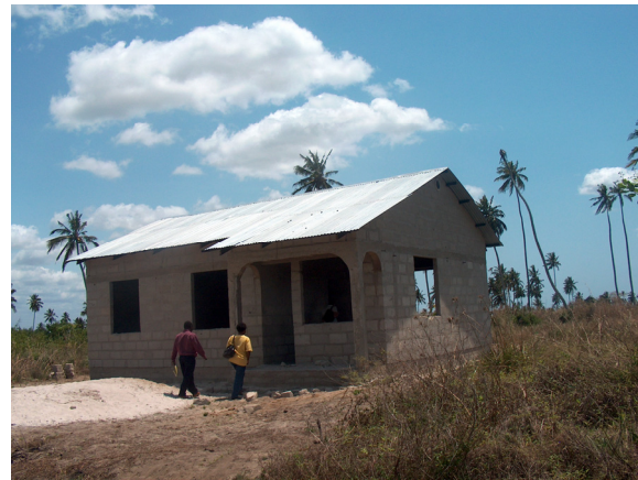
Fig. 2.11 Completed Shell, Demonstration House
