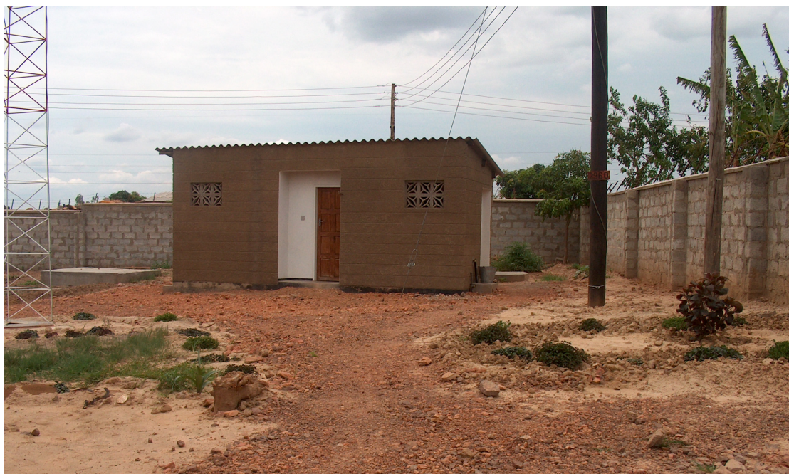
Fig. 2.4a Toilet Block for the Health Centre. Note the Solid Boundary
