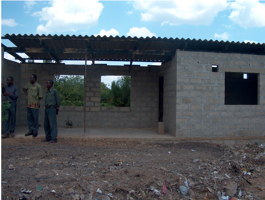
Fig. 2.2b Skills Training Centre under construction – Chazanga.
