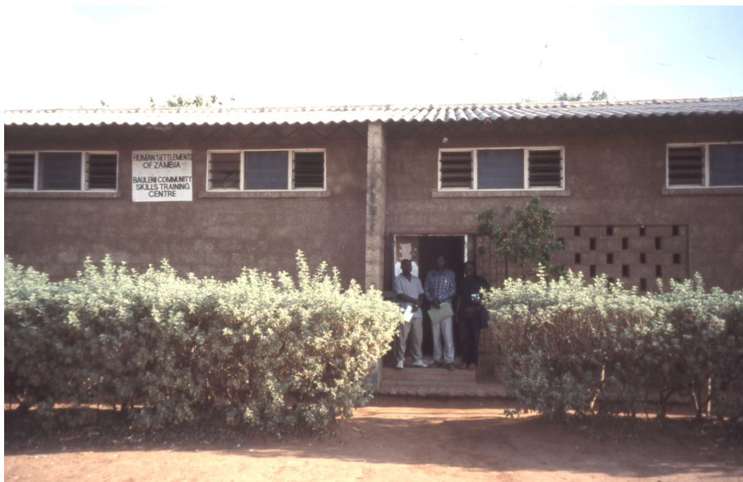
Fig. 3.4a Community centre and HUZA Office
