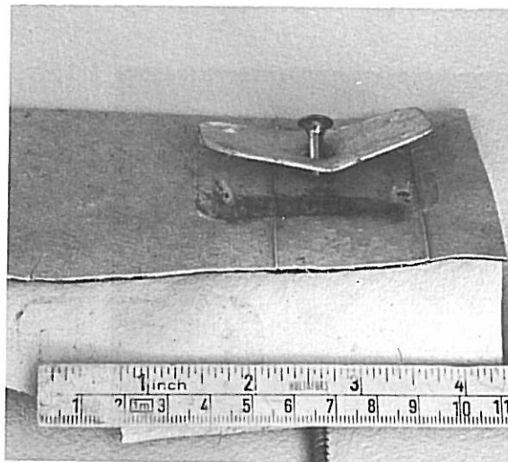
Photo 20 Roof III; fixing through two layers of membrane
