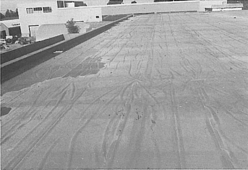
Photo 6. Homogeneous PVC membrane with folds over the whole surface.
