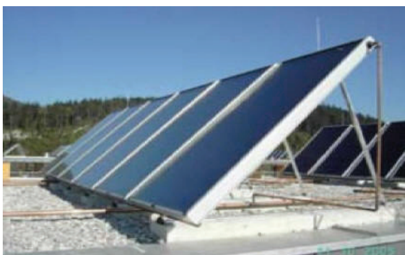
FIGUR 4-2 Takmontert solfangerpanel.
