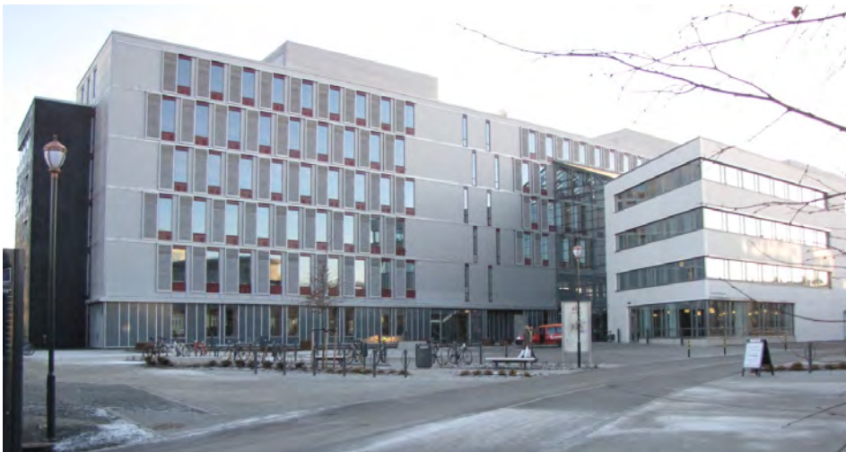
Figure 6 - entrance view of the building at Prof. Brochsgate 2 (ill. Rambøll Norge AS)
