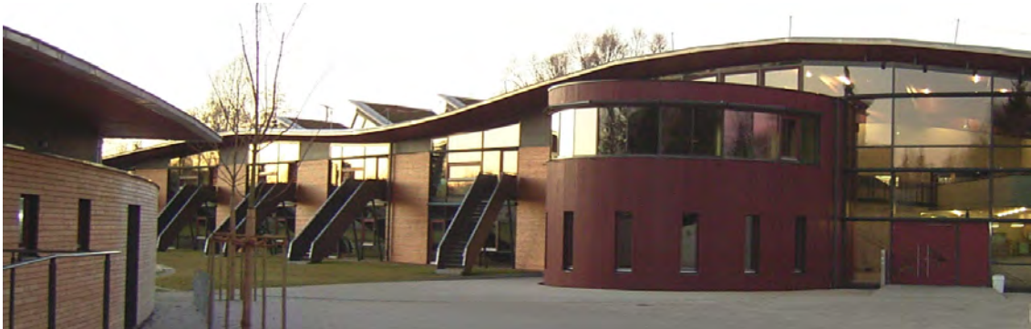
Fig. 1 View from the south – entrance and classrooms
