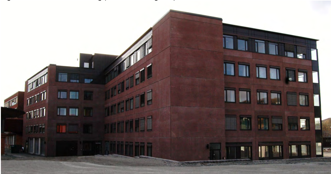
Figure 2 - facade office building (ill. Rambøll Norge AS)
