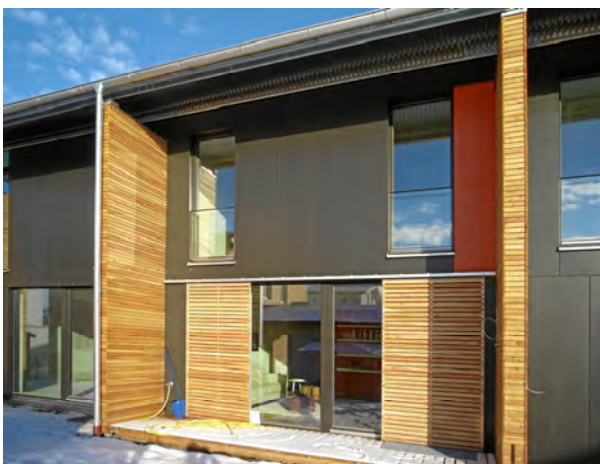
Fig. 6 View to the south
