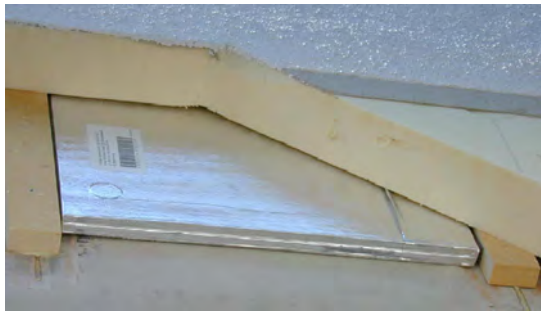
Fig. 3. VIP external insulation on a concrete wall (Pool 2009).
