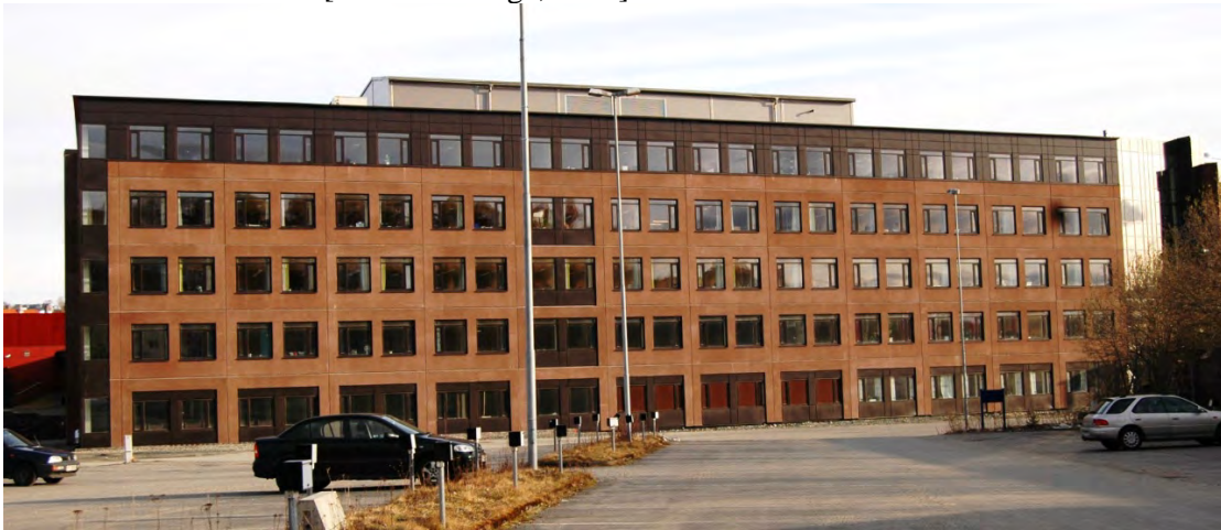
Figure 1 - Facade office building (ill. Rambøll Norge AS)
