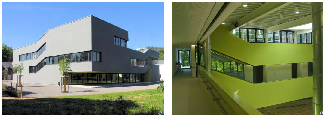
Fig. 2 Science College Overbach, Germany. Concrete façade with plastered insulation ( http://www.enob.info/de/neubau/projekt/details/science-college-im-bildungszentrum-overbach/ ).
