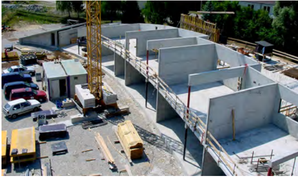
Fig. 4 View to the concrete construction
