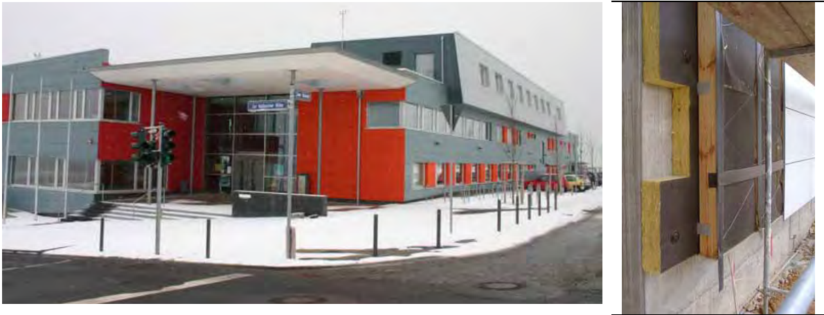
Fig. 3 Primary school and kindergarten Frankfurt-Riedberg, Germany. Concrete façade with curtain wall ( http://www.passiv.de/04_pub/Literatur/Riedberg/PH-Schule_Monitoring.pdf ).
