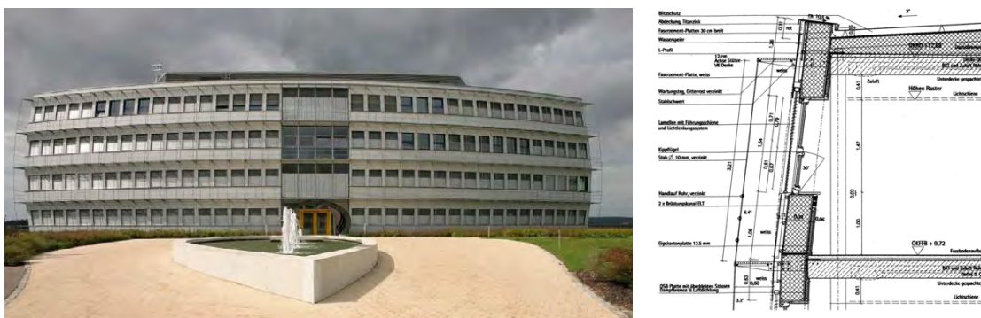
Fig. 1 Energon, office building in Ulm, Germany. Concrete in combination with wooden façade elements ( http://www.enob.info/de/neubau/projekt/details/passivbueroegebaeude-energon/ ).
