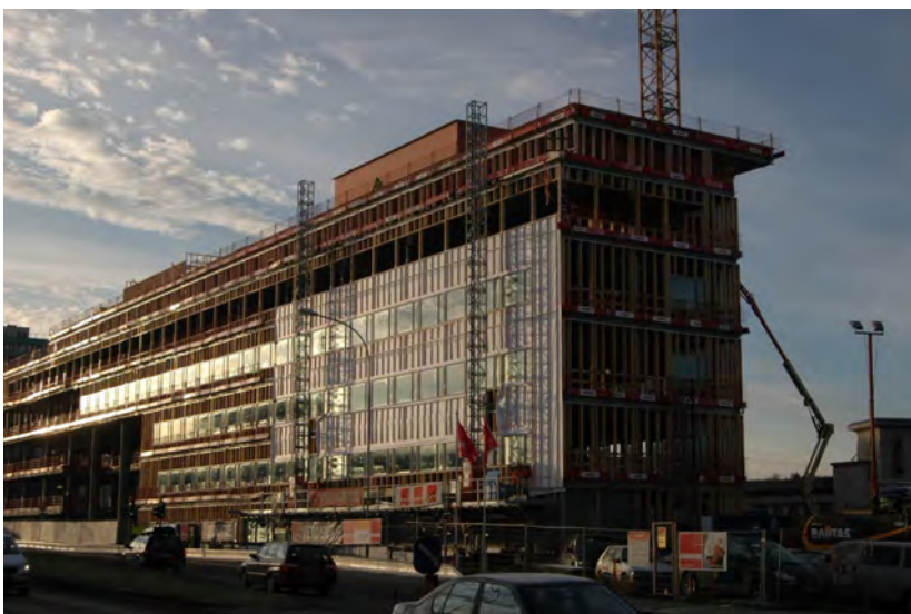
Figure 9 - office building prof. Brochgt. 2, timber framing facade (ill. Rambøll Norge AS)
