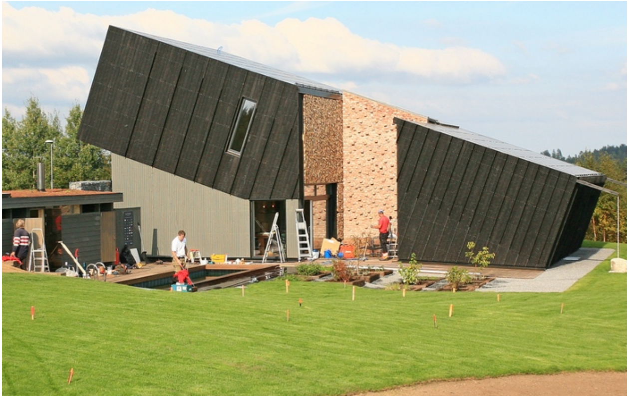
Figure 6.1 The Multikomfort house. Photo: Jon Østgård.
