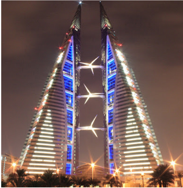
Figure 6 – Building augmented wind turbine, horizontal axis (World Trade Center, Bahrain). For more explanation see also Figure 13).
