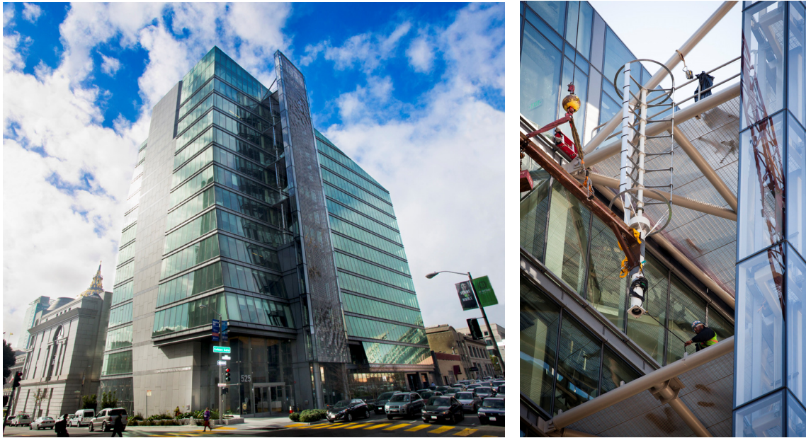
Figure 5 – Building integrated wind turbines with vertical axis (Public utility commission HQ, San Francisco)
