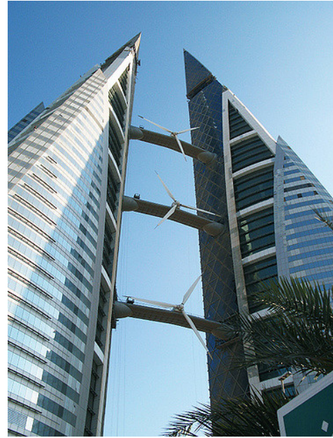
Figure 6 – Building augmented wind turbine, horizontal axis (World Trade Center, Bahrain). For more explanation see also Figure 13).
