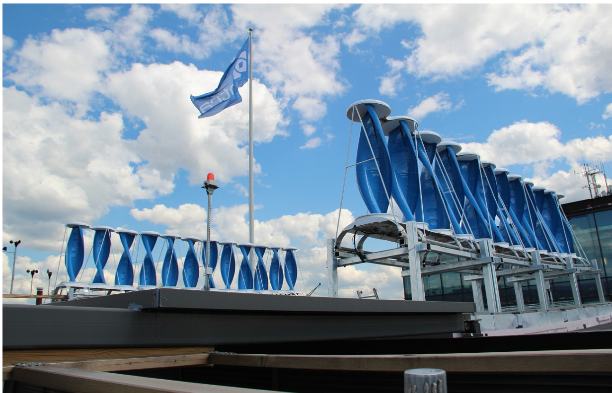
Figure 19 – Installation of wind turbines and wind measurement devices
