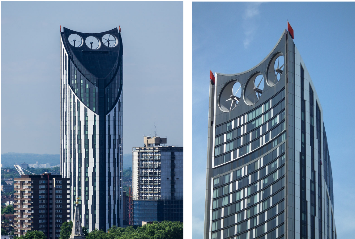
Figure 4 – Building integrated wind turbines with horizontal axis (Strata SE 1, London)
