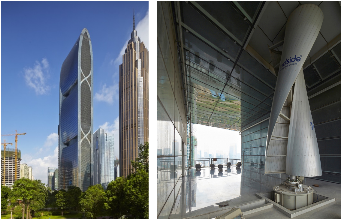
Figure 9 – Building augmented wind turbine (vertical axis) (Pearl River Tower, Guangzhou, China). For more explanation see also Figure 12.
