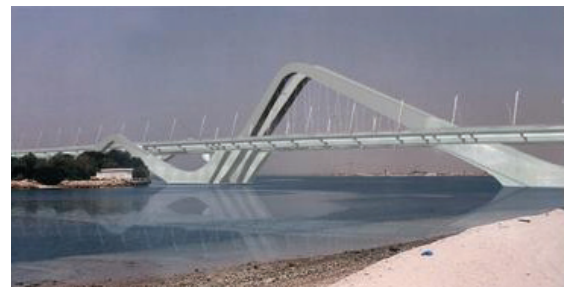
Figure 4-2: Sheik Zayed Bridge, Abu Dhabi. Lower part of supports are of reinforced concrete with steel type 1.4462 in the outer layer of reinforcement /32/
