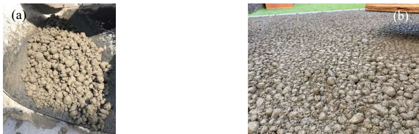
Figure 2 - Owacon concrete (a) fresh concrete before placement, (b) surface of placed Owacon after compaction.
