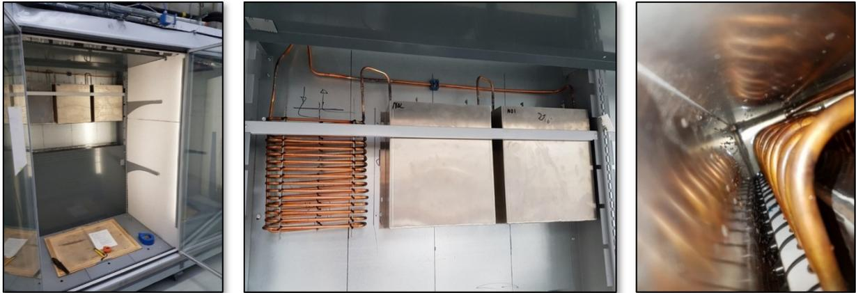
**Figure 3: Isolated middle section of a standard supermarket refrigerated display cabinet with three PCM-CTES containers, without wall panel between PCM-CTES containers and shelves (left); build-up of the PCM-CTES evaporator prototype (center) and refrigerant coil inside the PCM-CTES container (right).**
