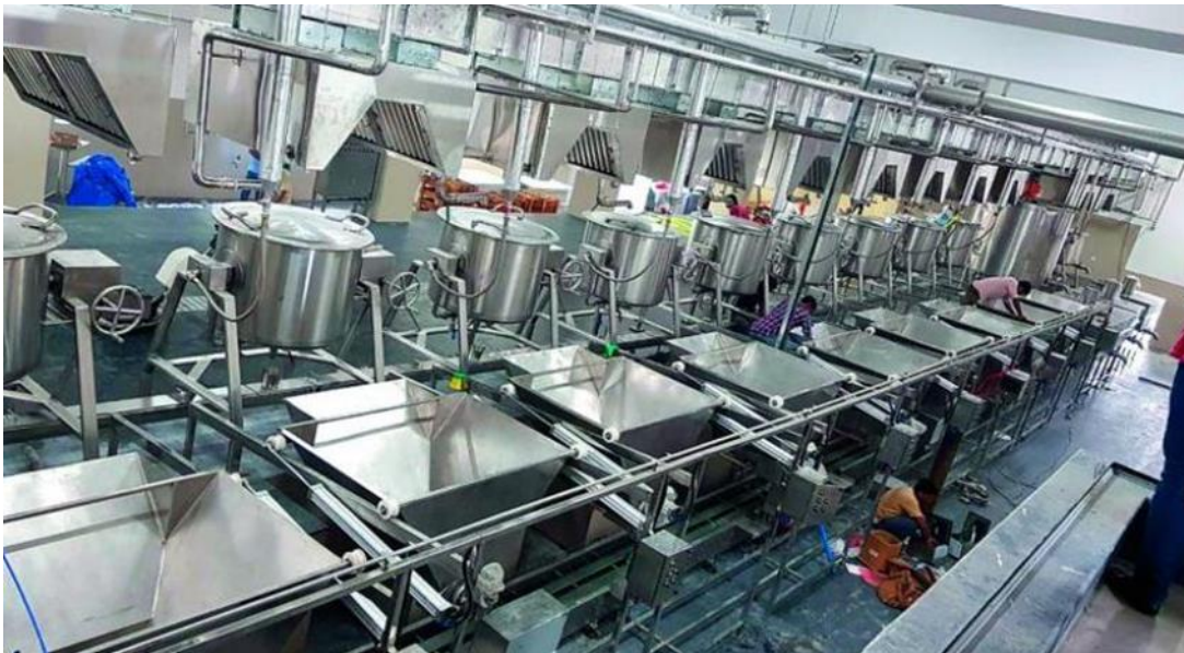
Figure 2-1: The centralised kitchen in Bengaluru
