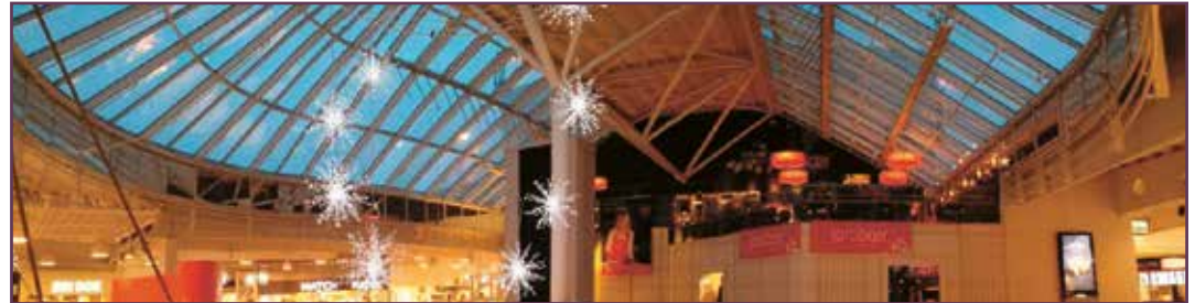
Figure 10.5 - City Syd demo case: skylights in the central atrium and the cafeteria located on the mezzanine below. Openable windows are present on both sides. Source: EURAC.
