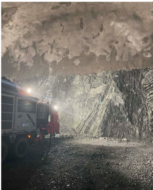
Figure 18. Photo from the end wall in one of the halls. The picture shows the rock support of the end wall in the roof and the upper part of the wall (Mørck et al., 2022).
