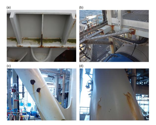
**FIGURE 3** Corrosion attacks on painted steel on offshore installation with different root causes. (a) Corrosion attacks initiating from edges; (b) galvanic corrosion around stainless steel welded into the structure; (c) poor pretreatment before paint application; (d) the paint is cracking and corrosion initiates in the cracks. [Color figure can be viewed at wileyonlinelibrary.com]
