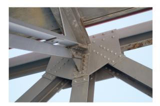
**FIGURE 9** Typical corrosion attacks on bolted thruss work on a coastal steel bridge protected with a TSZ duplex coating system. [Color figure can be viewed at wileyonlinelibrary.com]
