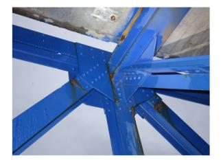
**FIGURE 7** Typical corrosion attacks on bolted truss work on a coastal steel bridge protected with a three-coat paint system. [Color figure can be viewed at wileyonlinelibrary.com]
