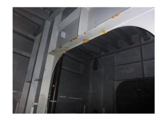
**FIGURE 5** Typical corrosion attacks in ballast water tank after 6 years in service. [Color figure can be viewed at wileyonlinelibrary.com]
