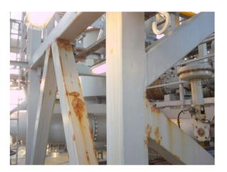
**FIGURE 2** Corrosion attacks on painted steel structure. Attacks typically initiate at welds and edges, but in this picture we also see attacks on flat surfaces, indicating that the film thickness is below specification. [Color figure can be viewed at wileyonlinelibrary.com]
