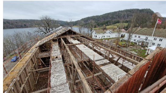
Figure 12. Nedre Sem Veidekke disassembling donor building (FutureBuilt)
