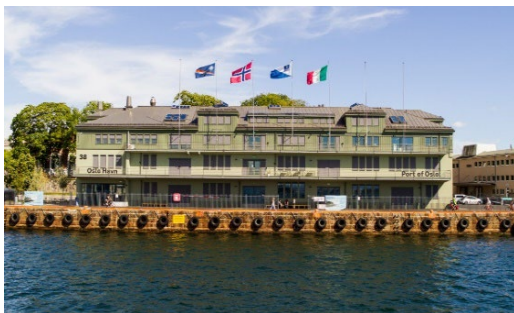
Figure 9. Skur 38 Oslo havn (FutureBuilt)
