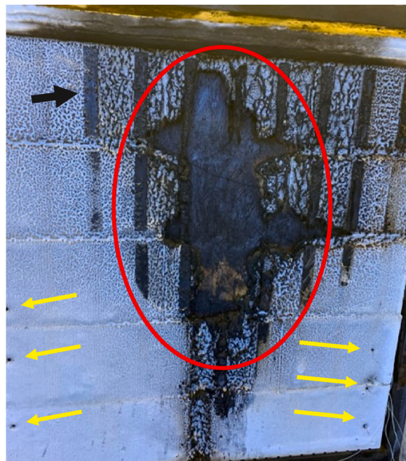
Fig. 21. Damage to the EPS insulation following Test 1 (a single layer of standard chipboard, test duration: 10 min).
