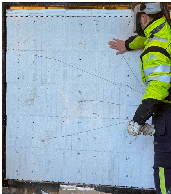
Fig. 26. Damage to the EPS insulation following Test 6 (two layers of standard gypsum board, test duration: 15 min). The lines on the specimen are pencil marks showing the location of the thermocouples.
