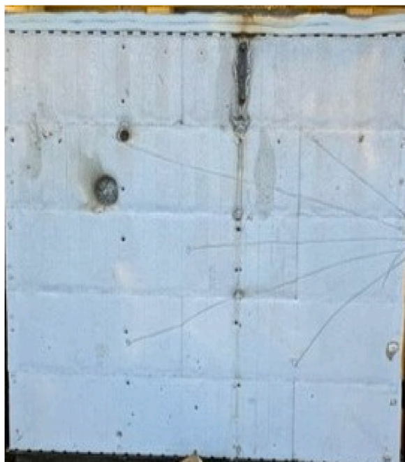
Fig. 27. Damage to the EPS insulation following Test 7 (a single layer of gypsum board, test duration 10 min).
