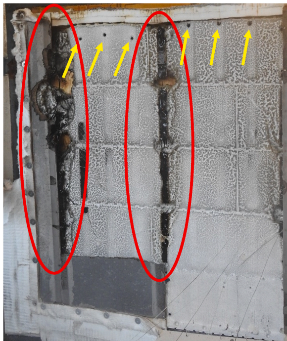
Fig. 24. Damage to EPS insulation following Test 4 (a single layer of gypsum fibre board, test duration: 15 min).
