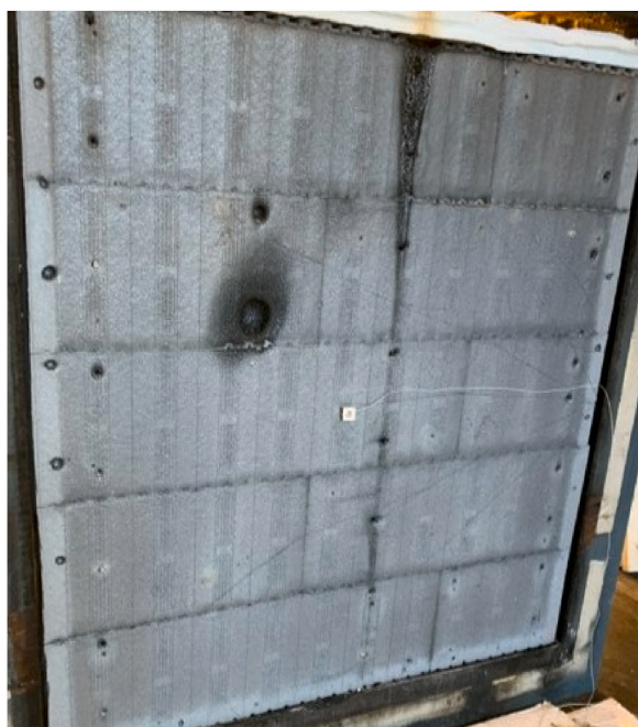
Fig. 28. Damage to the EPS insulation following Test 8 (fire-retardant EPS covered by a single layer of gypsum board, test duration 10 min).
